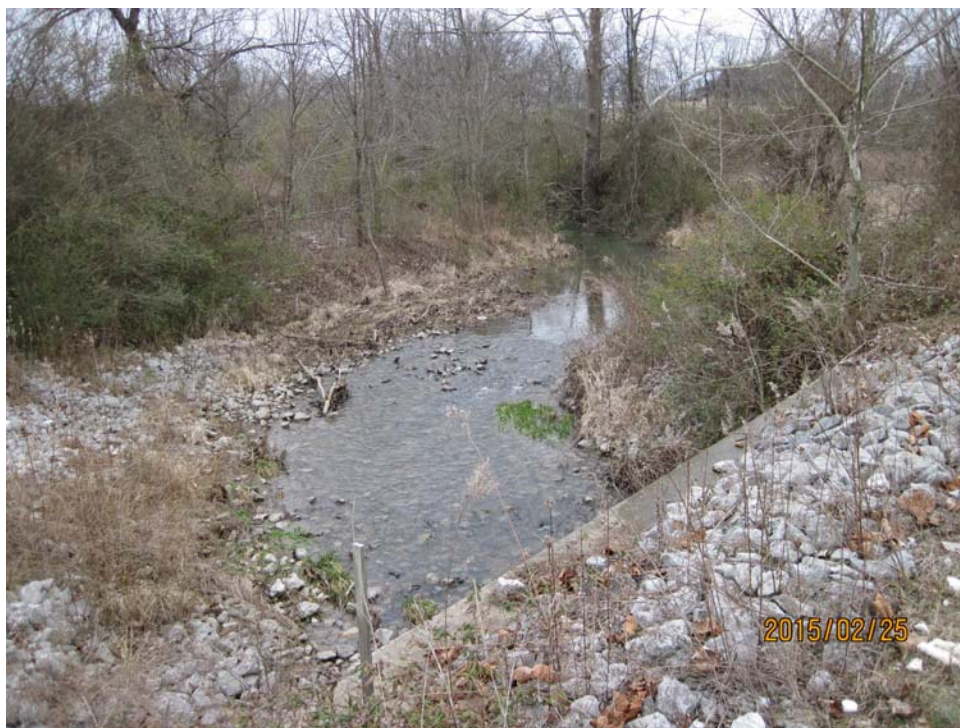
View upstream from existing box culvert on STR-2, Station 125+80R.
