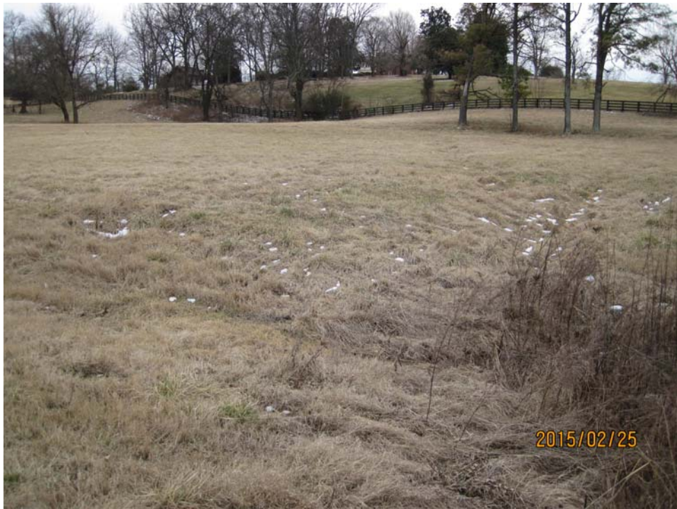
Grass swales on east side of SR-6 that direct precipitation runoff into the box culvert at Station 100+30R. No aquatic feature at this location.
