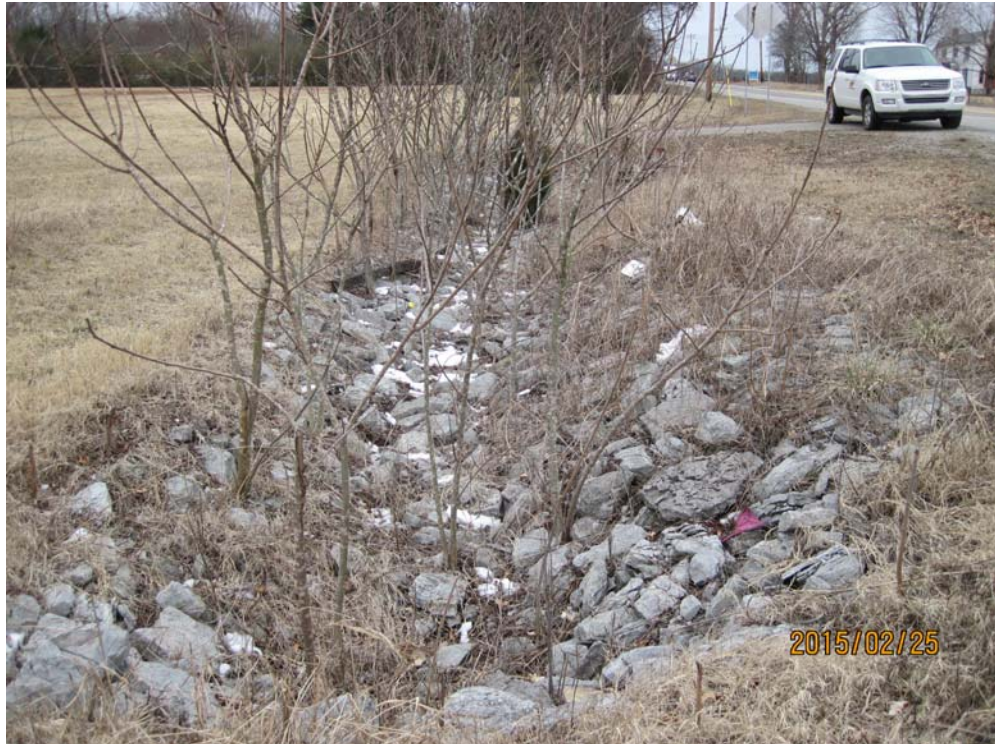
Riprap stormwater ditch; view up-gradient (south) from Station 121+50R.
