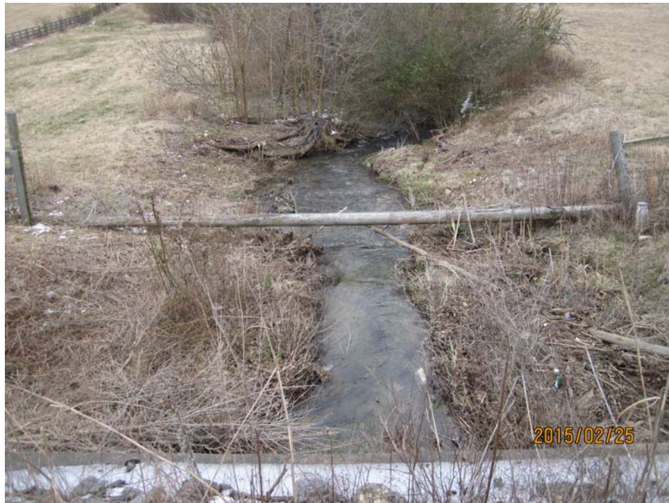
View downstream from existing box culvert on STR-2, Station 125+80L.
