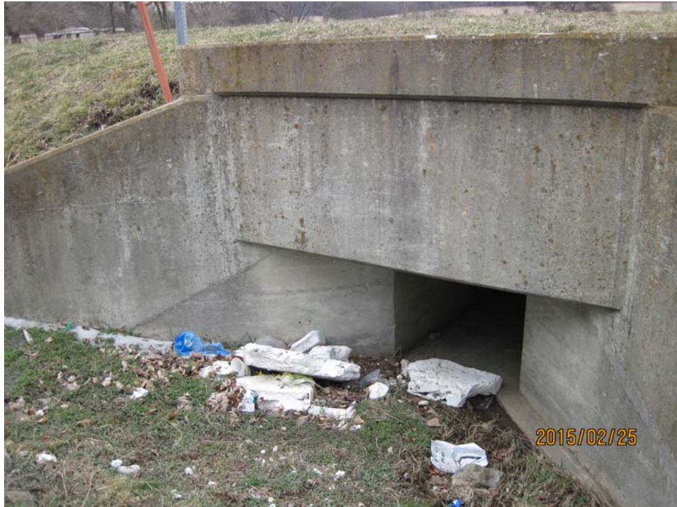
Inlet of box culvert at Station 100+30R (No aquatic feature here).
