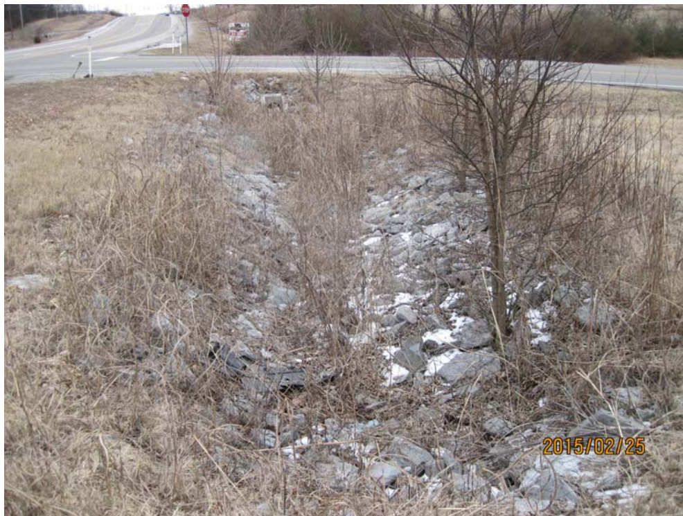
View down-gradient in riprap stormwater ditch from Station 121+60R. No aquatic feature at this location.
