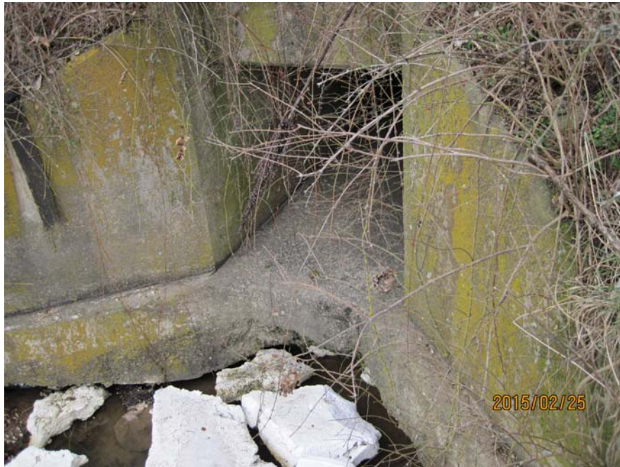
Culvert outlet at Station 100+30L, and start of STR-1 (Stream Source under concrete).
